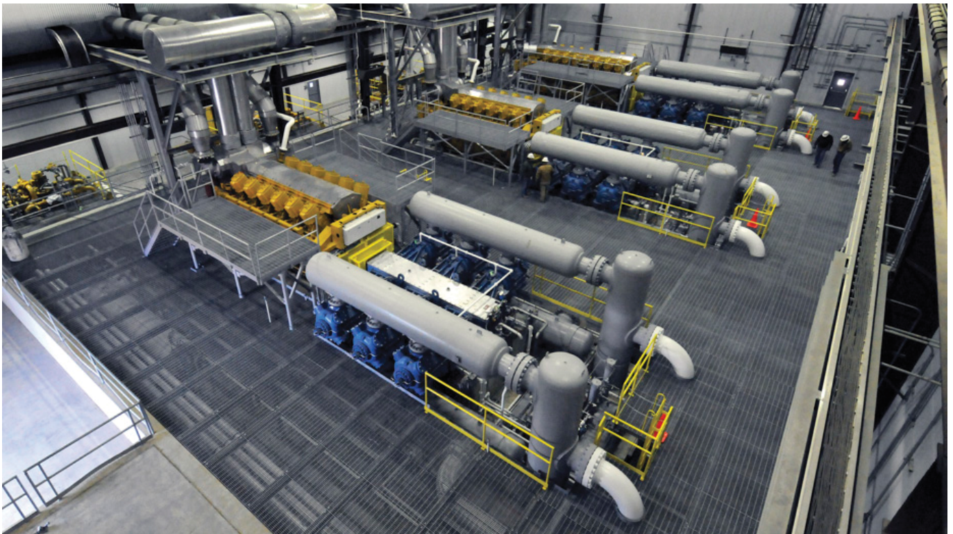
REX gas pipeline in the USA. Compressor package with the KBU/6 driven by gas engine 6 MW.
