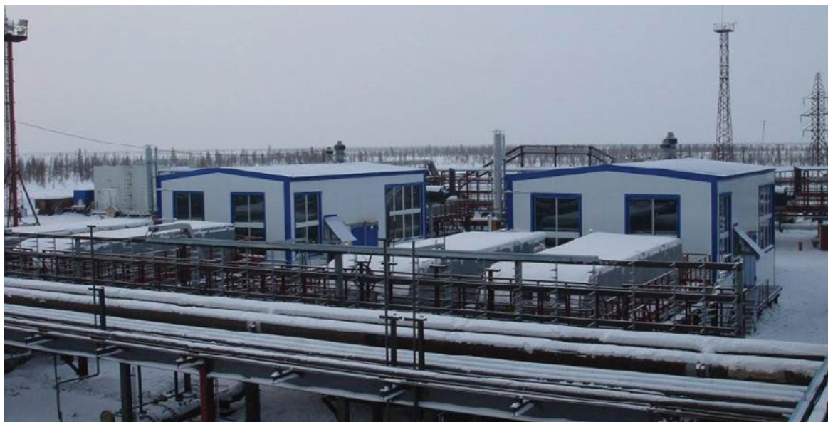
NOVATEK - TARKOSSALENNEFTEGAZ. Compressor package with Ariel JGC/6-2 driven by gas engines 3.6 MW.
