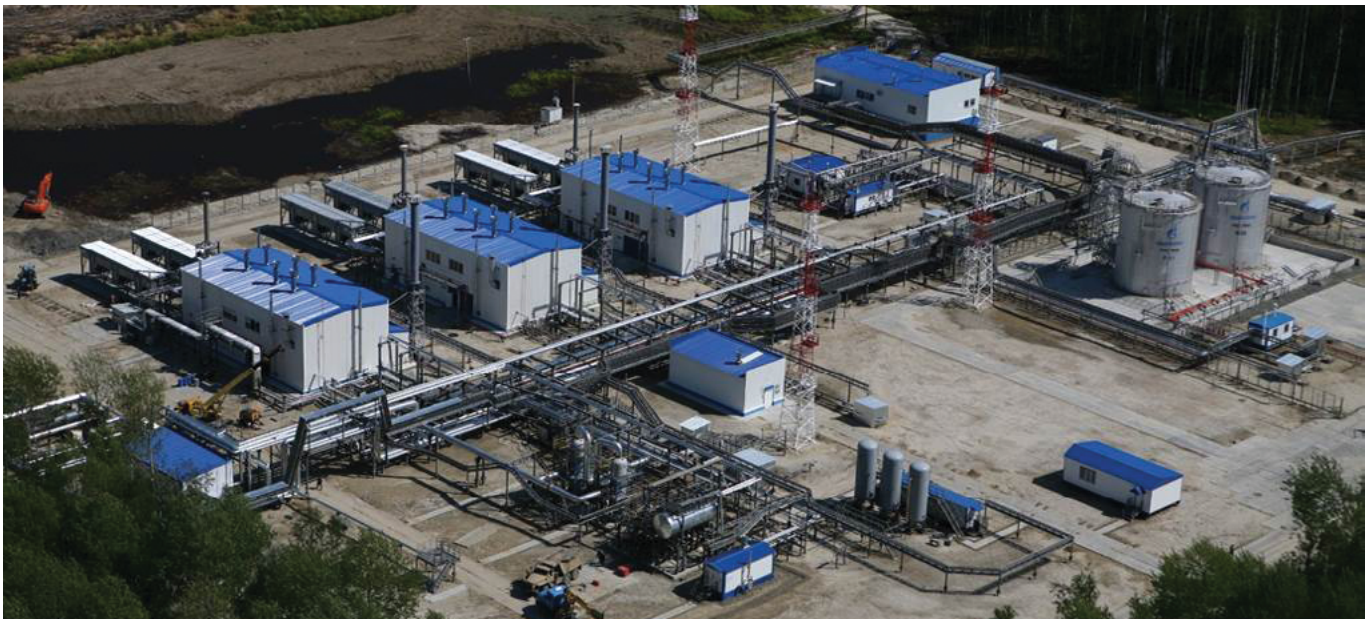
Tomskgazprom, Kazanskaya - 1. Three compressor packages with Ariel compressors JGZ/6-3 driven by gas engines 3.6 MW.
