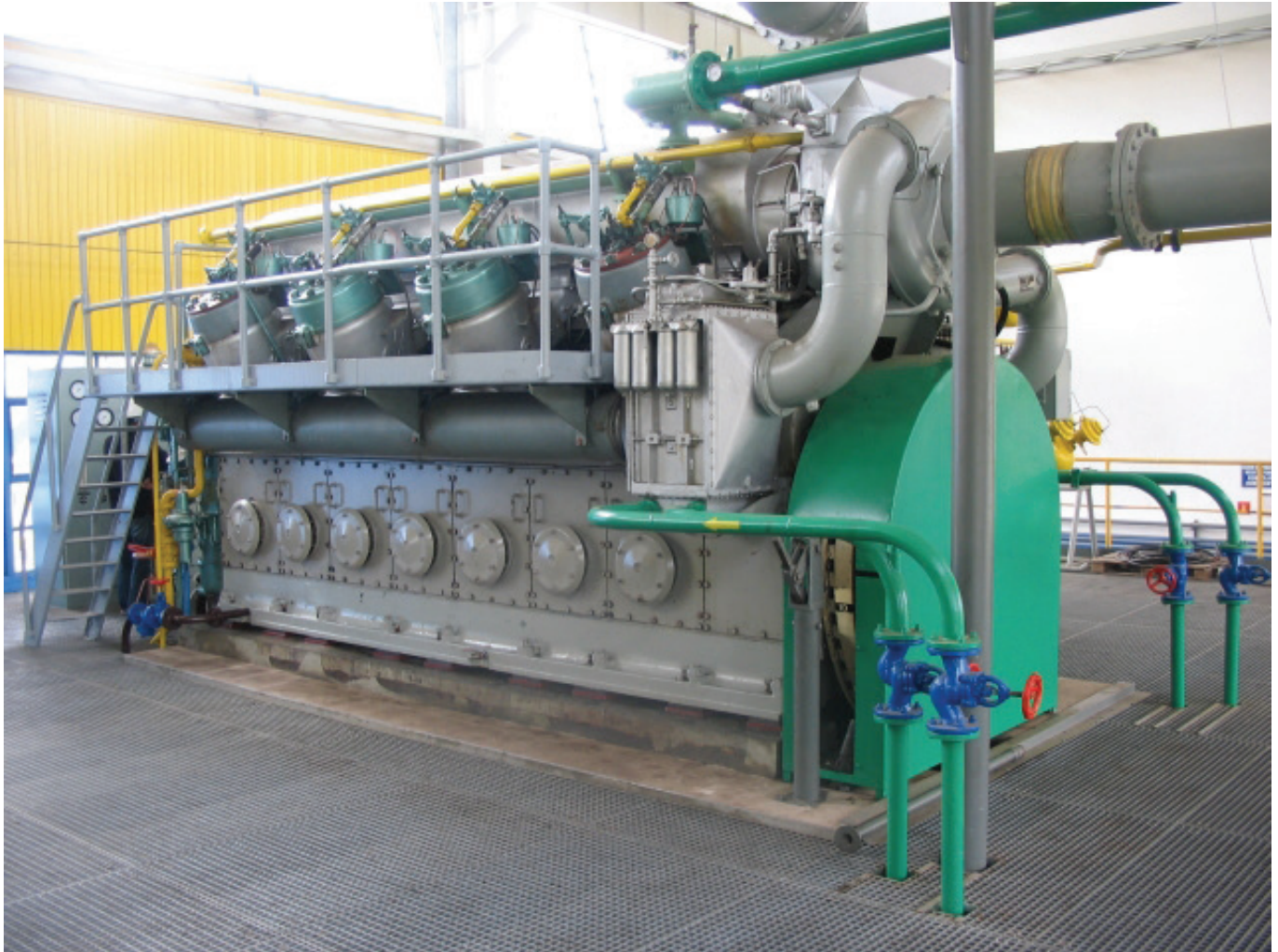
Gas engine LSV 16 at the power station
