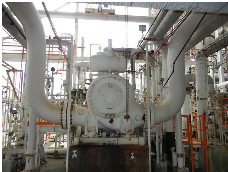
Centrifugal compressor RFB 24 driven by Elliot turbine rated 4800 hp at 7550 rpm.
